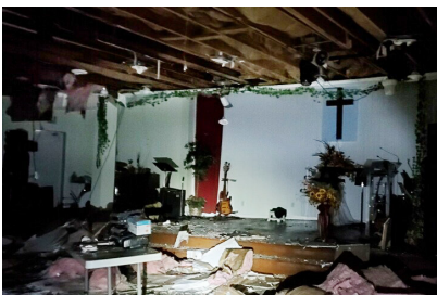
The building of Vietnamese Baptist Church is a total loss after it was burned during unrest in Philadelphia. (Photo from Pastor Philip Pham)
