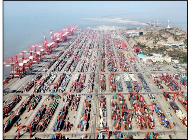
Yangshan Deep Water Port
